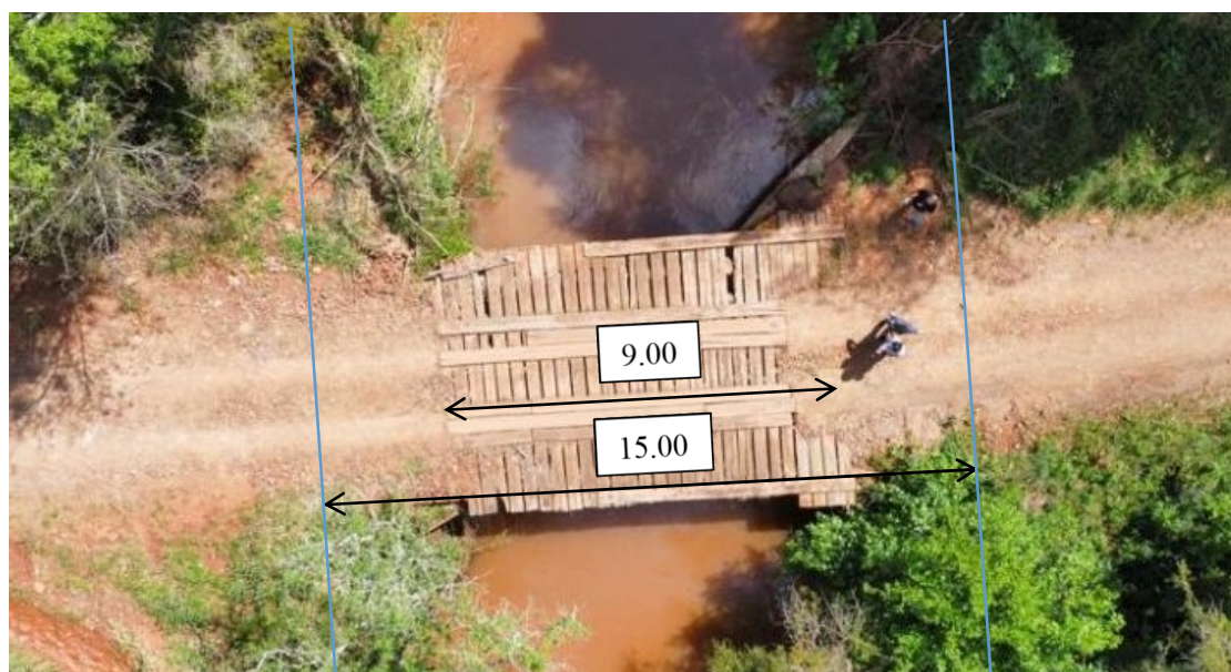
Vistoria in loco 29/09/2023.
