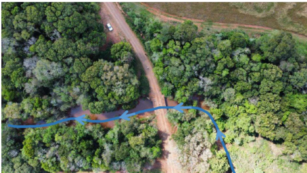
Vistoria in loco , 29/09/2023.
