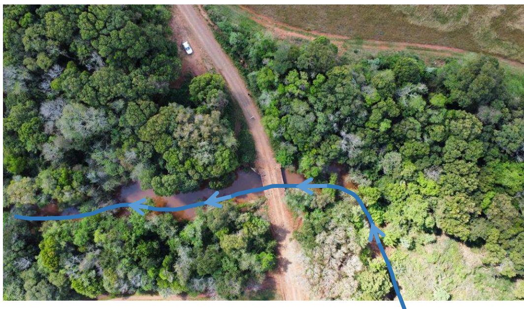
Vistoria in loco 29/09/2023.
